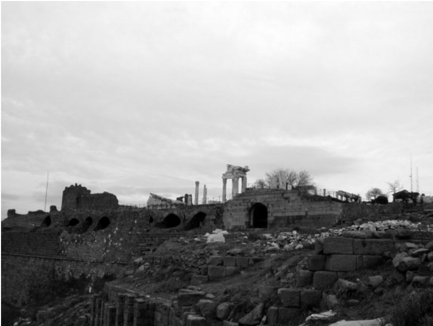
Fig. 2. Vaulted chambers supporting the Trajaneum platform.
